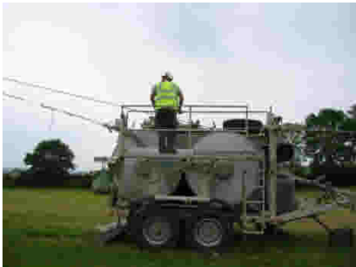
Illustration 5.8: Winching machine for stringing operation.
