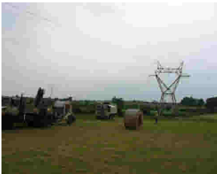
Illustration 5.9: Stringing location during operation.
